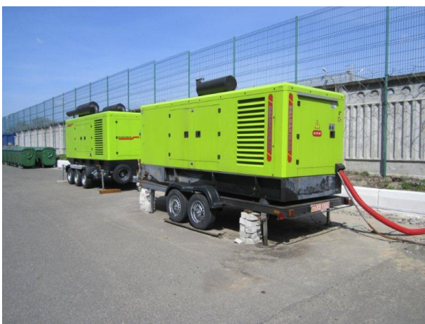
Photo No.3. Diesel-generators of reserve capacity
